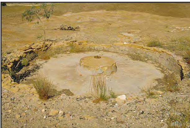
Remains of a circular buddle used to concentrate slimes from jigging machines. (Photo 43614)
