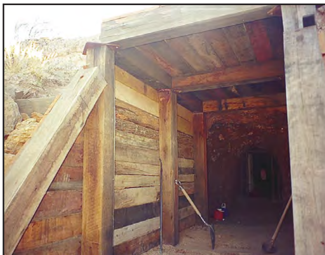
Re-timbering the miner's adit. (Photo 44296)
